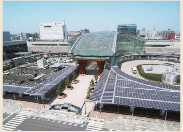
JR Kanazawa Motenashi Dome (above ground)
