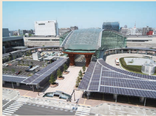
JR Kanazawa Motenashi Dome (above ground)
